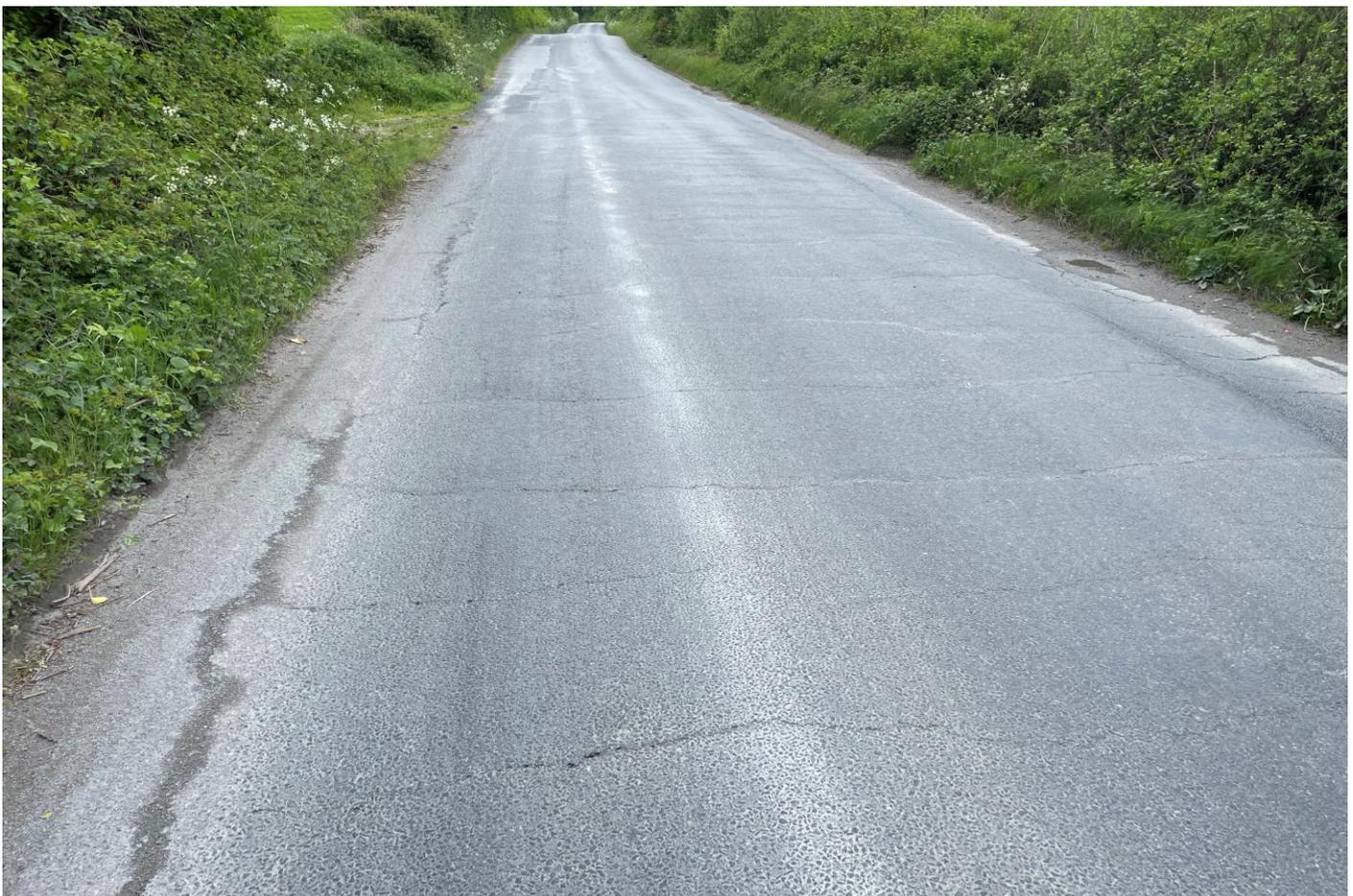
**Picture D11: Section C – Edge Repairs and surface distortion ~ Chainage 750**
