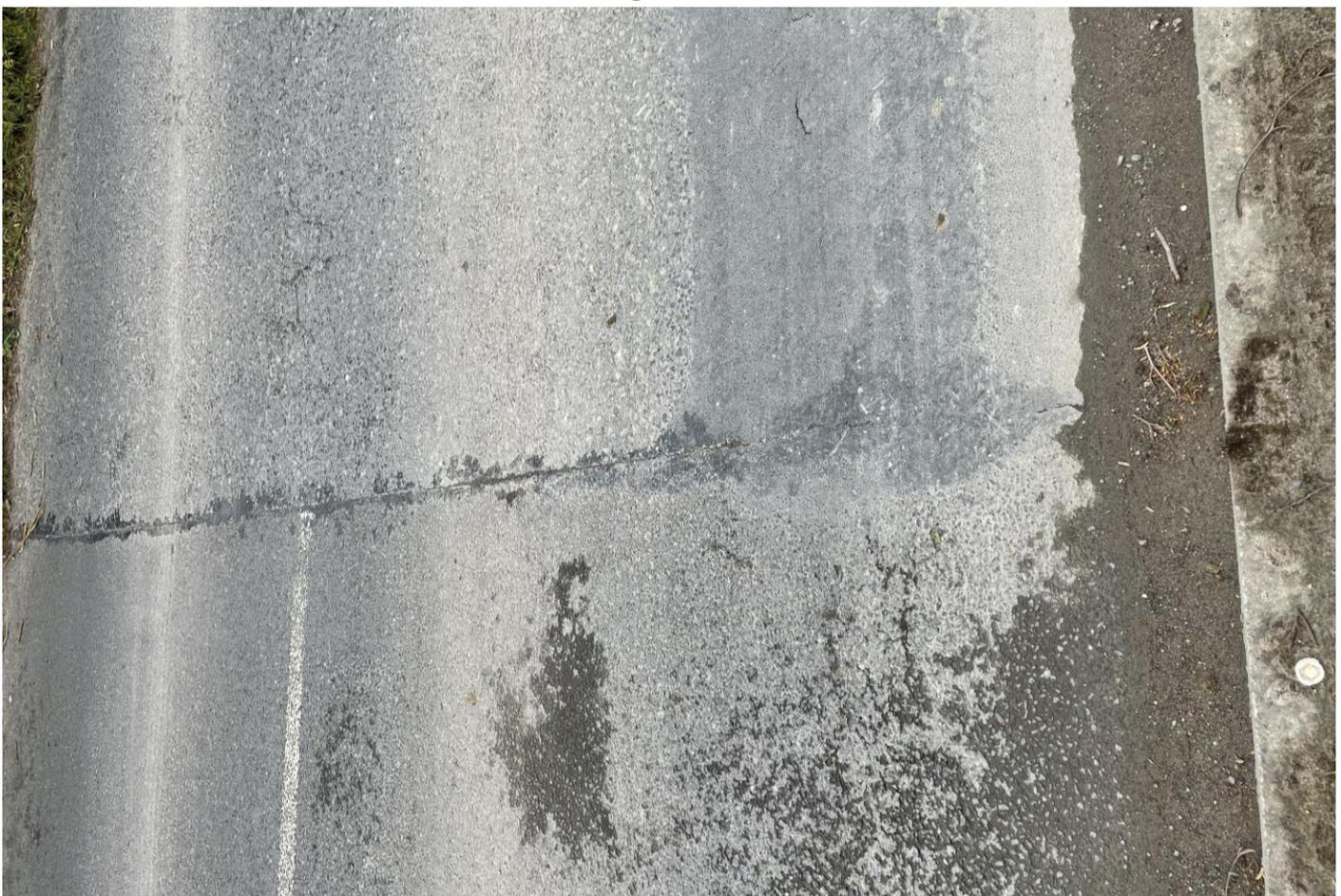
**Picture D7: Section B – Patching in good repair**
