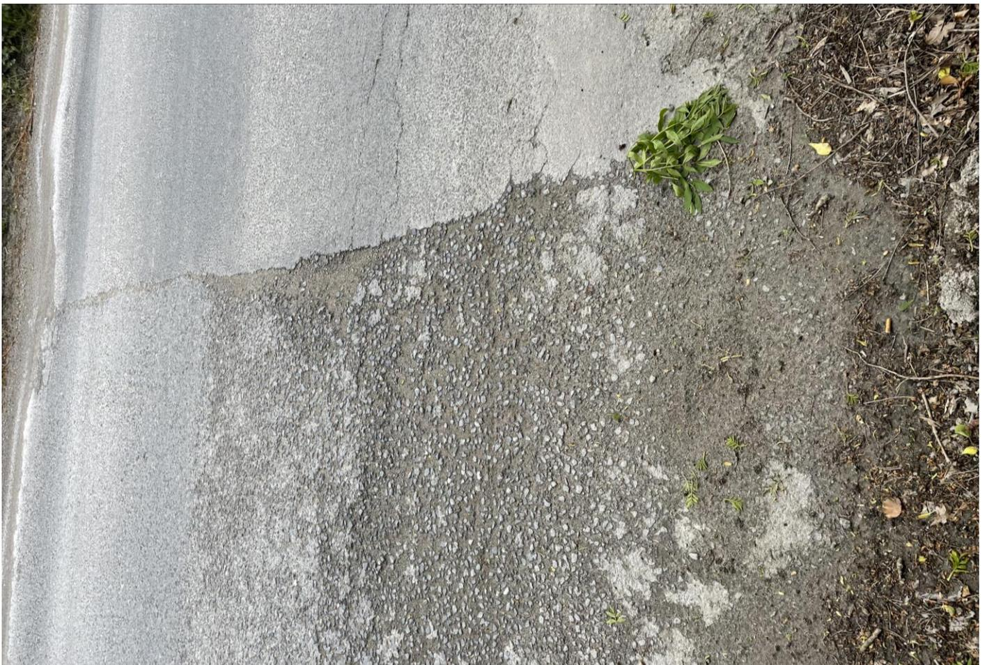
**Picture D9: Section C – Edge Damage, patching surface distortion ~ Chainage 450**
