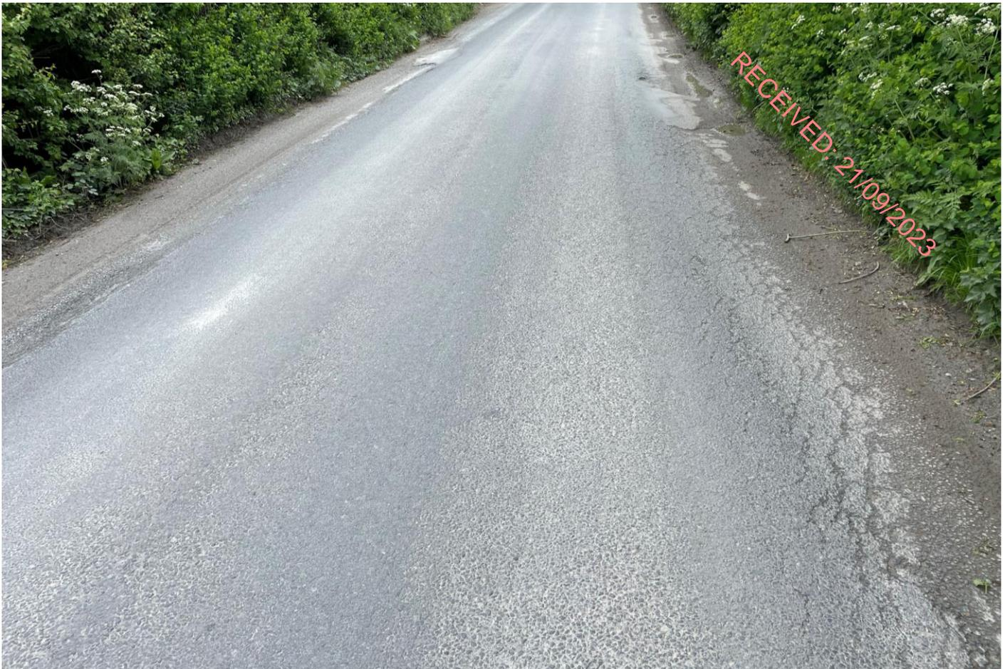
**Picture D10: Section C – Cracking and Surface Distortion ~ Chainage 700**
