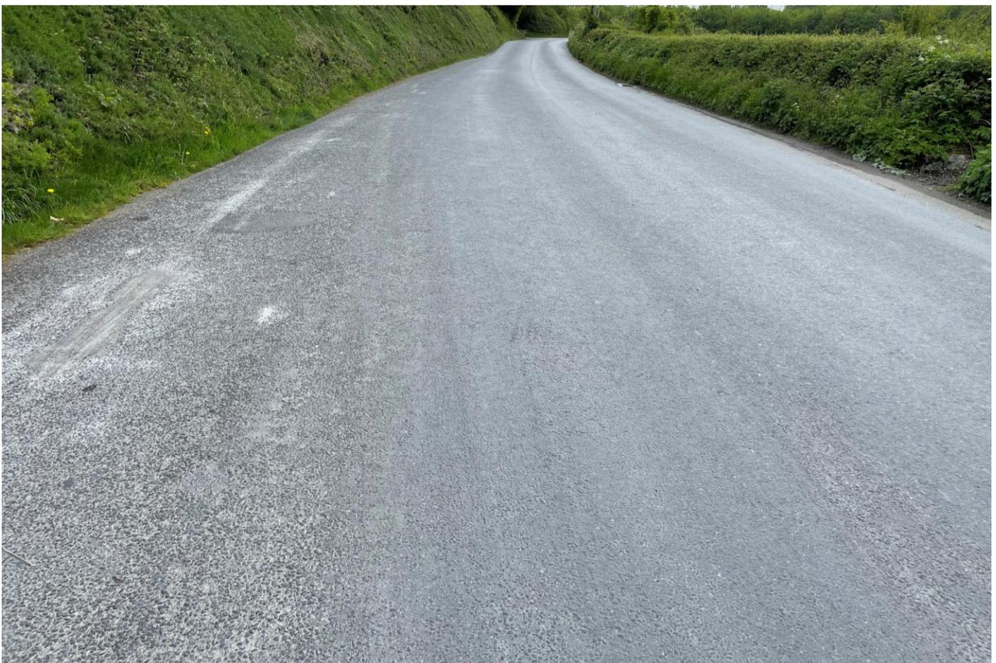
**Picture D15: Section D, Some edge damage and surface distortion, bleeding in wheel-tracks**
