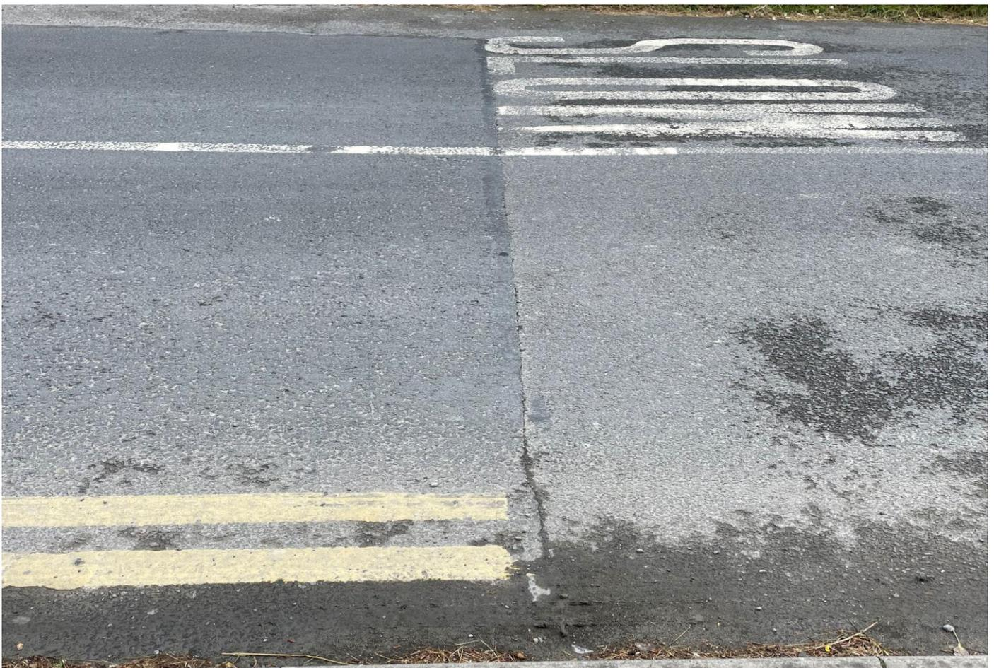
**Picture D3: Section A – Chainage 40, some cracking in wheeltracks**
