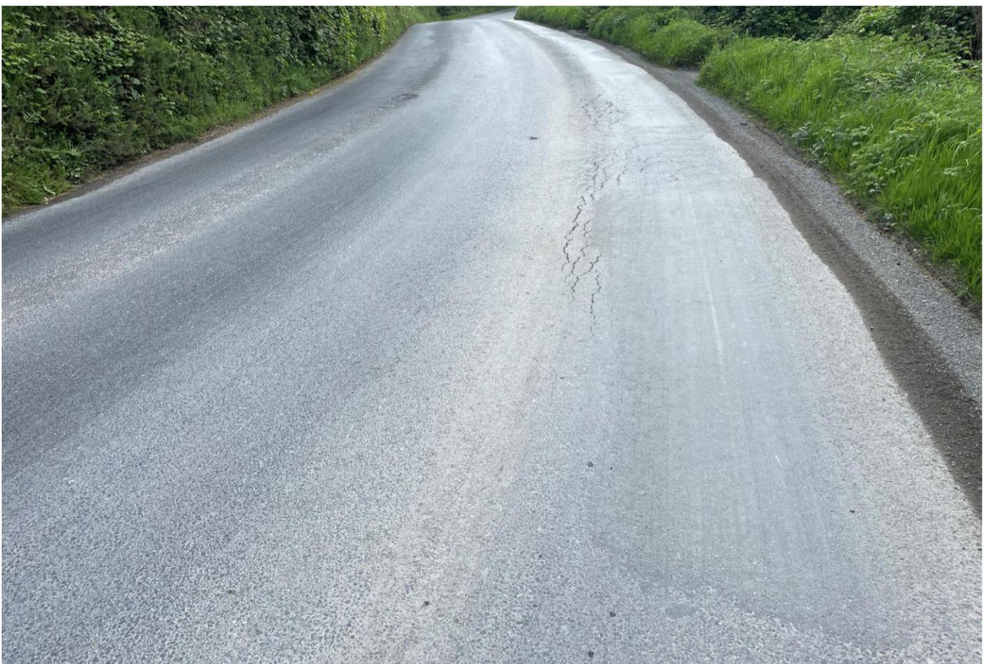
**Picture D17: Section D – Some cracking and distortion**
