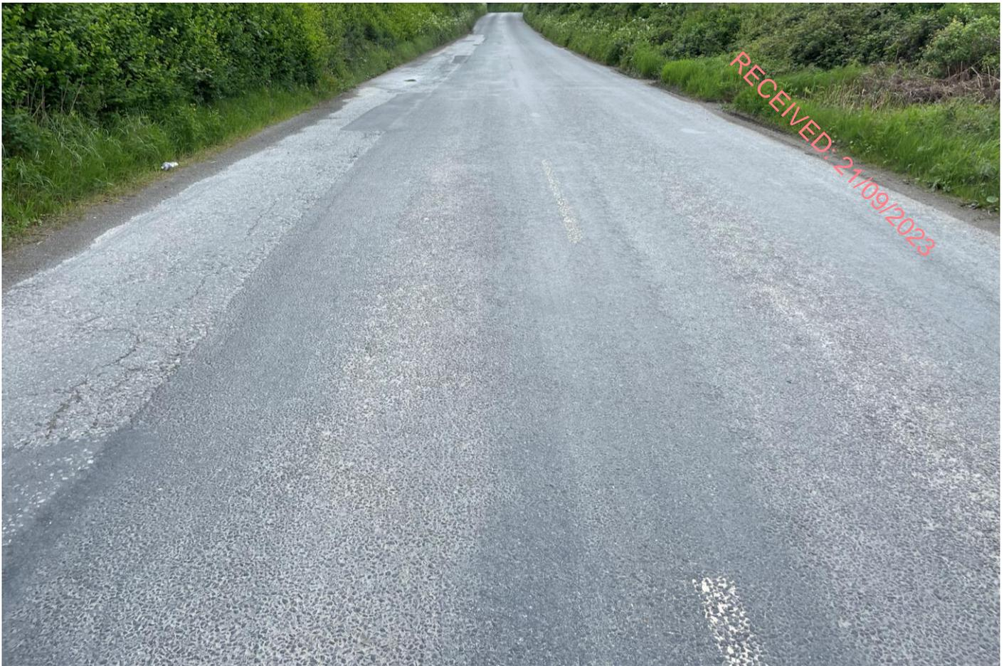
**Picture D12: Section C – Edge Damage and repairs ~ Chainage 1000**
