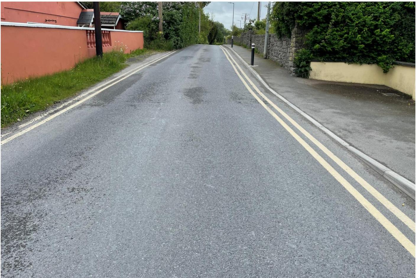
**Picture D5: Section A Chainage 140 – Good surface with Antiskid and Ramp**
